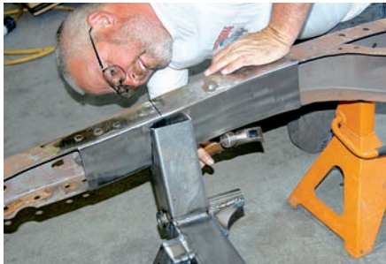
8) The crossmember was installed and it was a tight fit. A few hammer whacks were necessary to get the centerlines to match up.
