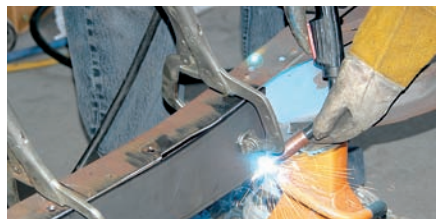
6) O'Bryant decided that it would be better to use a pair of hand clamps to secure the boxing plate before the welding was done. He started by tack-welding the section to the frame at the front and rear.
