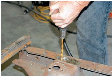
2) Using a 3/8-inch drill, the rivets were drilled to remove the shanks.
