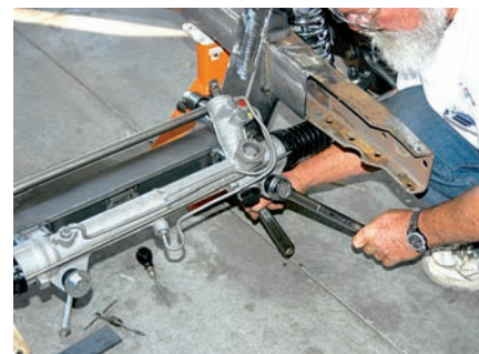
26) The rack-and-pinion unit was reinstalled and then it was tightened with a pair of 15/16-inch wrenches.
