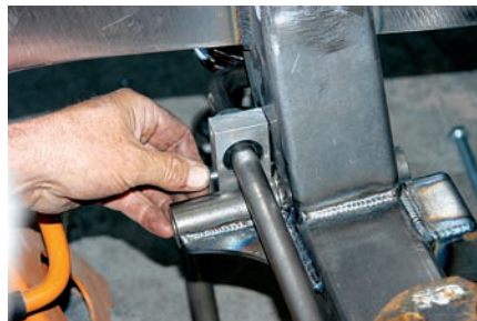
13) The Swaybar block was bolted to the crossmember on the bottom, and when it was in place, the upper bolt hole was drilled and tapped. Doing it this way ensures that the bolt holes will line up perfectly.
